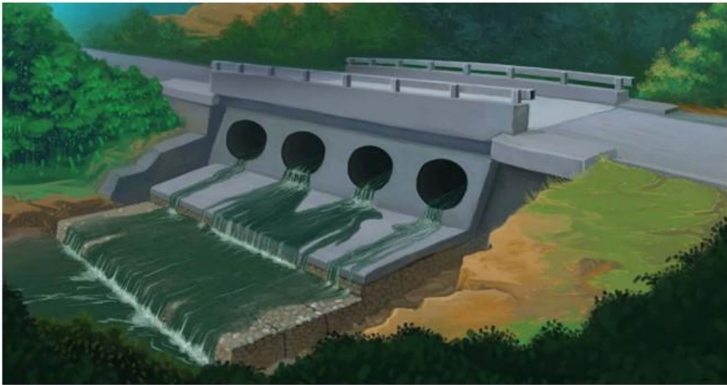
Picture: Outlet of water crossing structure
